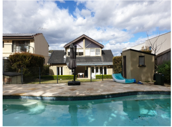
View from the rear of the property showing high hedge, high privacy fence and existing toilet to be removed
