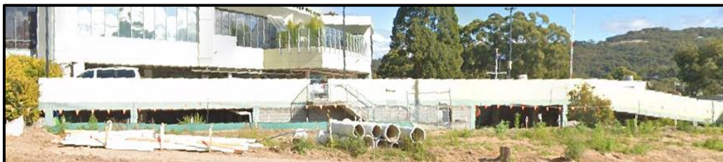
Figure 3: View of carpark area along Mona Vale Road frontage prior to extension of the external wall as an acoustic barrier (Source: Google maps – December 2021) NB: foreground works are Mona Vale Road upgrades
