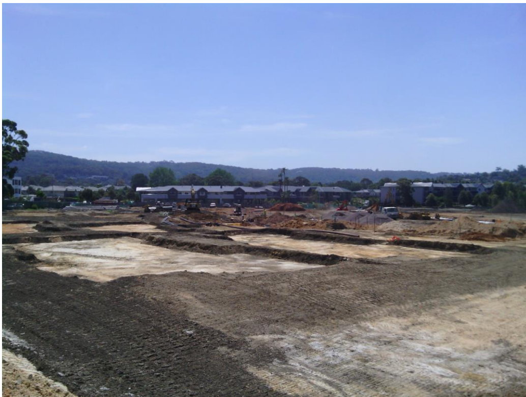
Plate 4. View of construction site to the west
