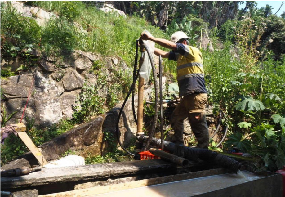
Photo 5: Drilling Bore 03 with portable equipment
