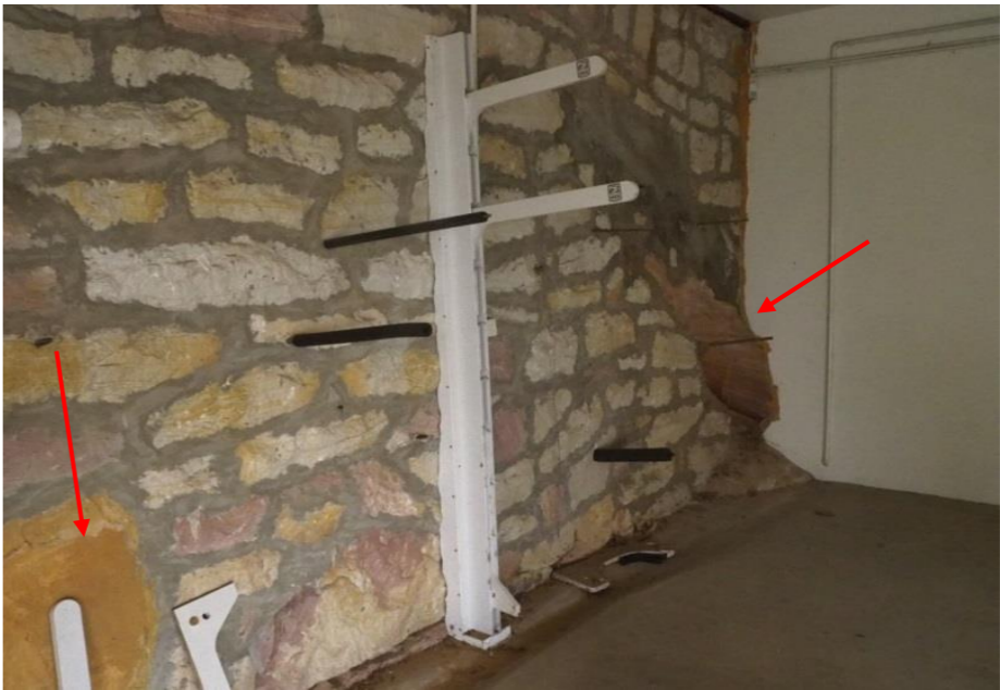
Photo 6: Detached sandstone boulders ('floaters') visible in rear garage wall
