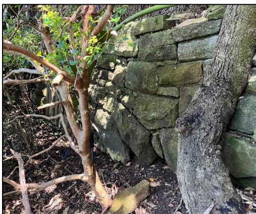
Photograph 3 and 4: View of slight bulging of the retaining wall supporting the Serpentine easement and minor settlement of steps
