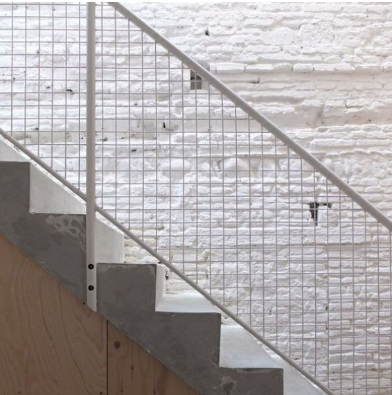
Precedent: Steel mesh balustrade & pool fence. To comply with AS3959-2009 & AS1932-2012 (MSC)
