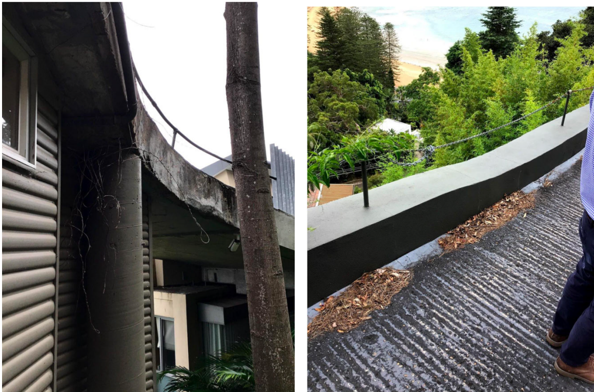
Source: Taylor Consulting Engineers, Private driveway – right of way on 6 Mitchell Road
