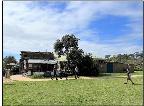
Photograph 2: The rear of the surf club, as viewed from the north-west
