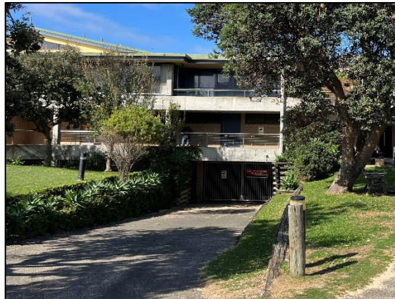
Photograph 16: Vehicular entrance, as viewed from the north-east
