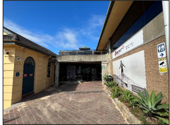
Photograph 15: Main building entrance, as viewed from the north-east
