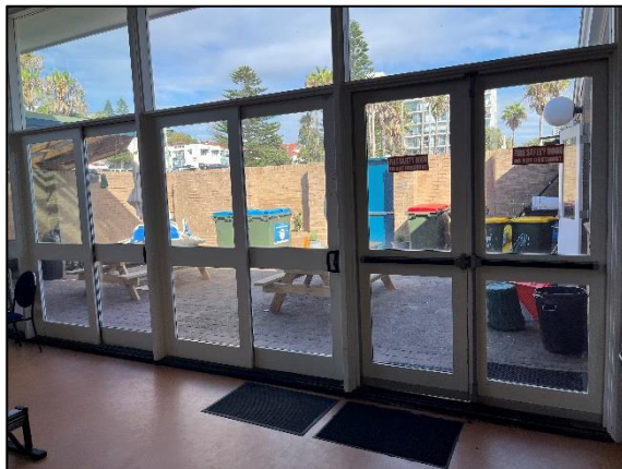
Photograph 10: The rear terrace, as viewed from the recreation hall
