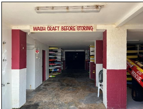
Photograph 4: Storage facilities within the basement
