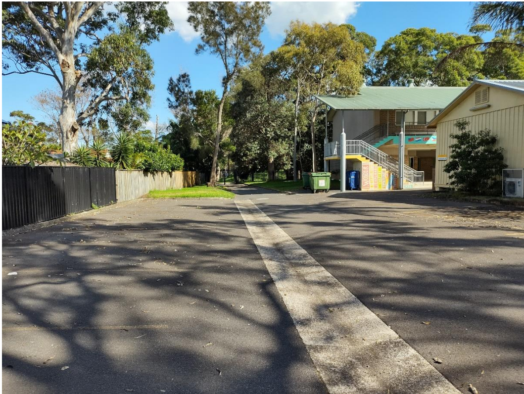
Photo 8: NNPS – Looking at driveway entry off Namona Street and eastern side of Building V.
