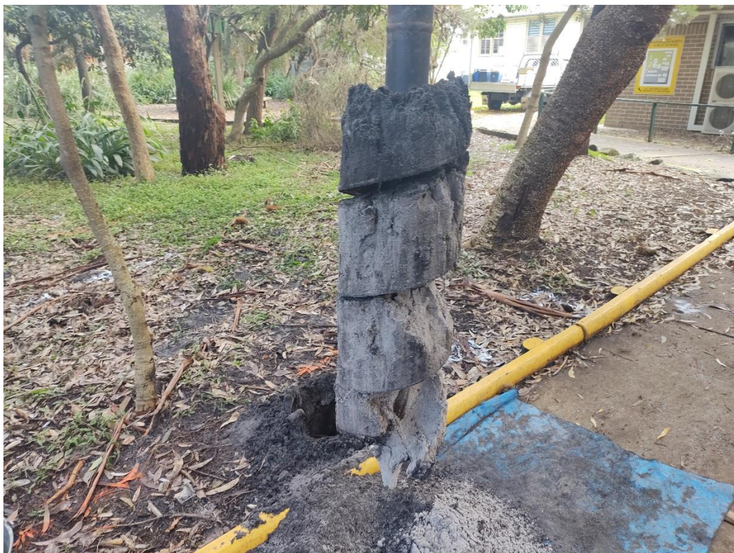
Photo 10: NNPS – Typical borehole returns
