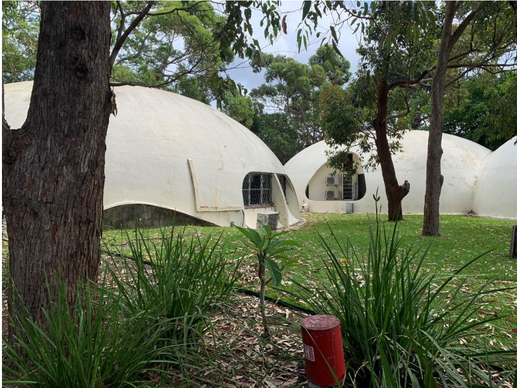
Photo 1: NNPS – Northern side of bini-dome building
