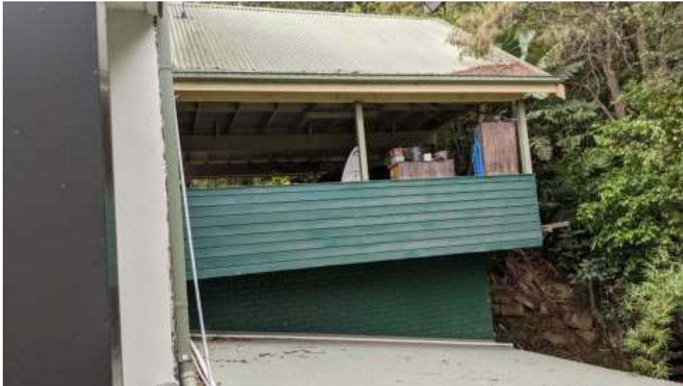
Looking at area of proposed addition from existing ground floor balcony
