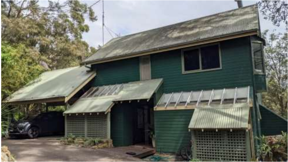
Looking at residence from driveway
