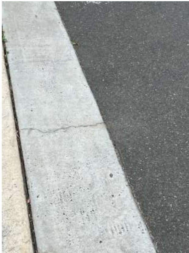
Figure 10 – Crack is evident to the layback outside 63 Warriewood Road Warriewood.
