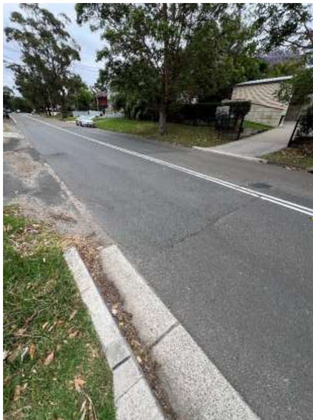
Figure 48 – Crack is evident to the road outside 49 Warriewood Road Warriewood.
