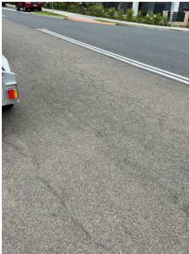
Figure 130 – Crack is evident to the road outside 82 Warriewood Road Warriewood.
