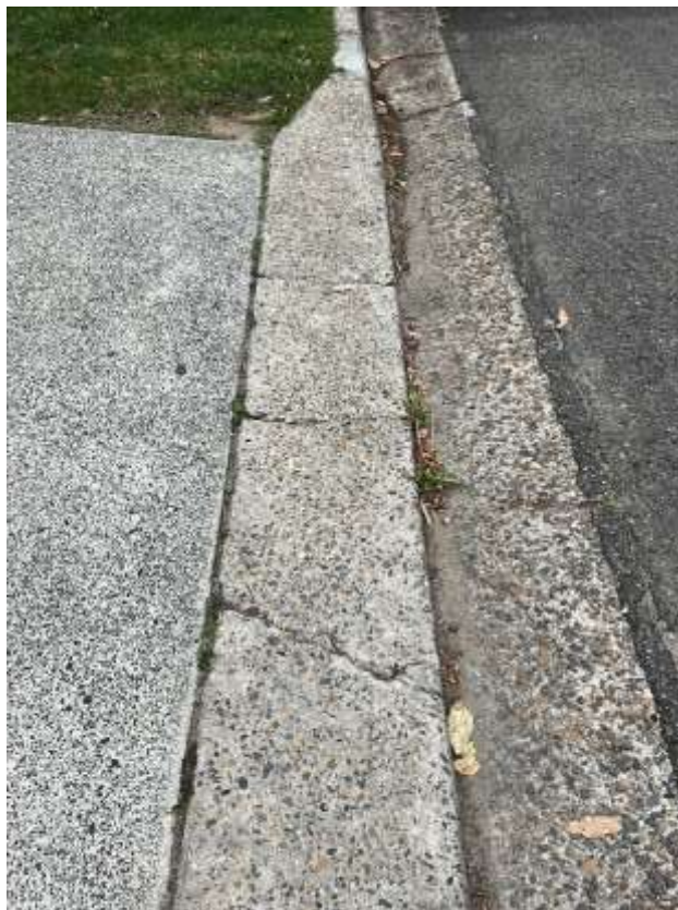
Figure 66 – Crack is evident to the layback outside 92 Warriewood Road Warriewood.
