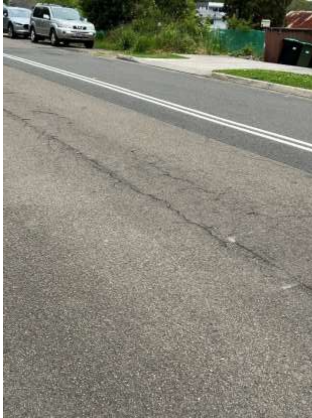
Figure 57 – Crack is evident to the road outside 92 Warriewood Road Warriewood.
