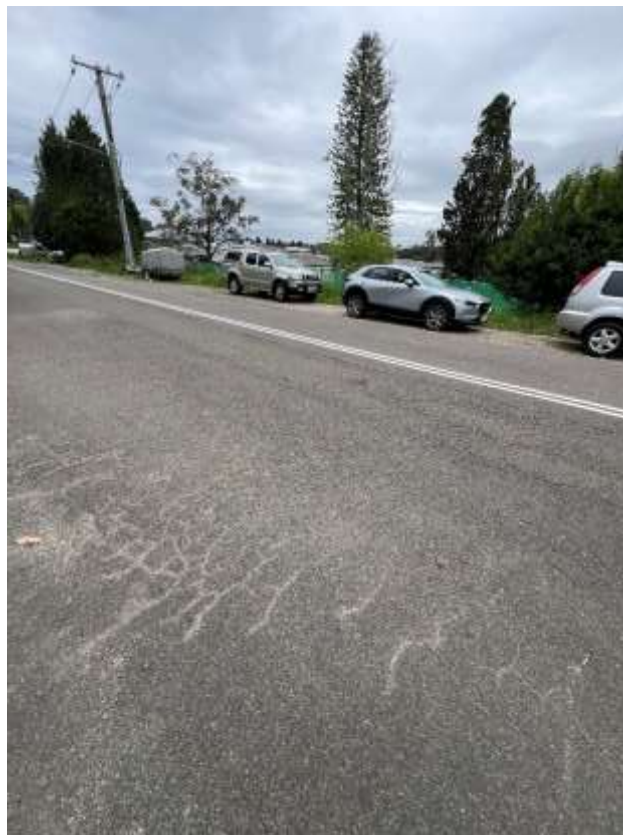
Figure 72 – Crack is evident to the road outside 92 Warriewood Road Warriewood.
