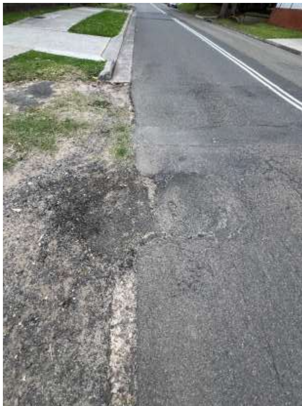
Figure 36 – Crack is evident to the road outside 49 Warriewood Road Warriewood.
