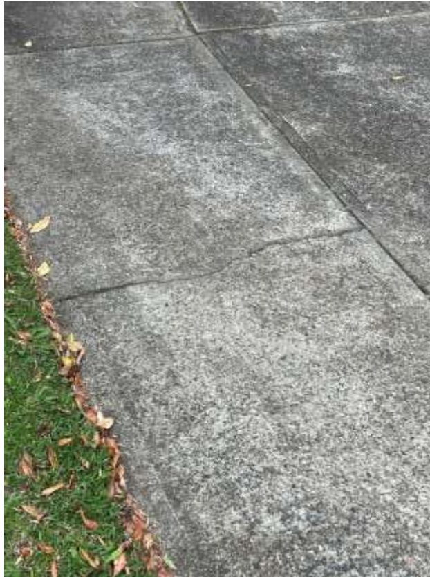
Figure 85 – Crack is evident to the driveway outside 88 Warriewood Road Warriewood.
