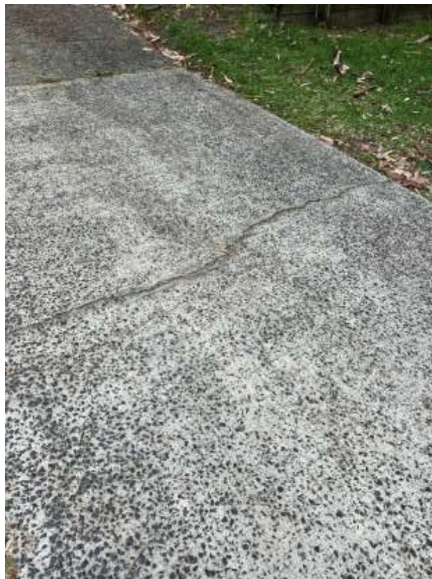
Figure 104 – Crack is evident to the driveway outside 86 Warriewood Road Warriewood.
