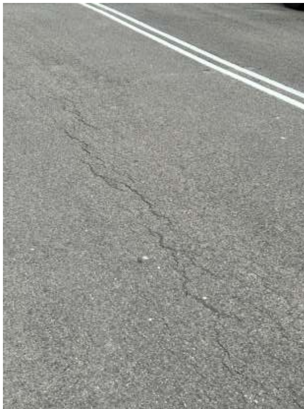
Figure 34 – Crack is evident to the road outside 45A Warriewood Road Warriewood.
