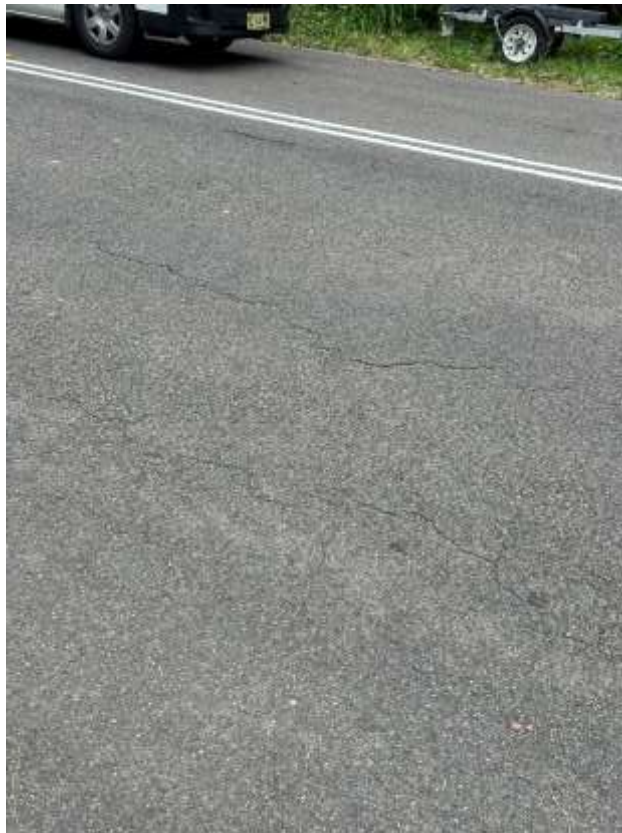
Figure 102 – Crack is evident to the road outside 86 Warriewood Road Warriewood.
