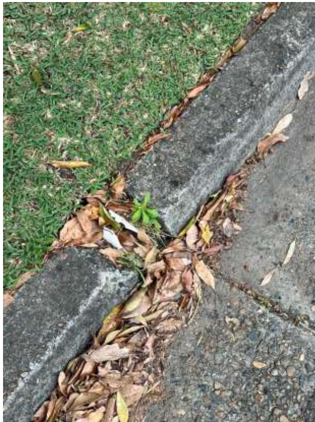
Figure 90 – Crack is evident to the kerb outside 86 Warriewood Road Warriewood.
