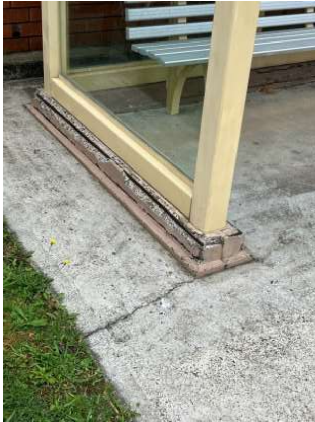
Figure 59 – Crack is evident to the concrete at bus stop.
