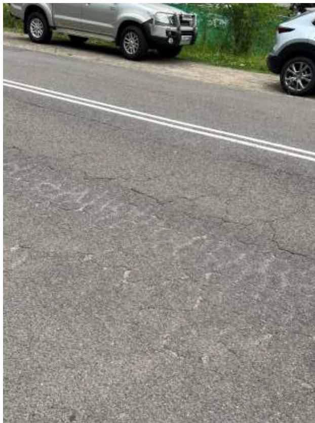
Figure 74 – Crack is evident to the road outside 90 Warriewood Road Warriewood.
