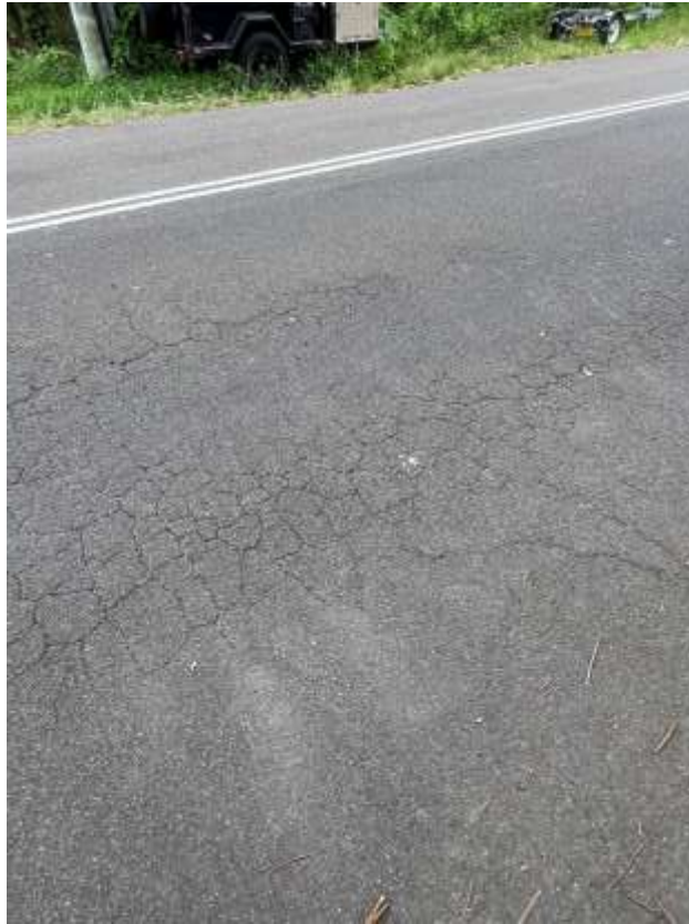
Figure 113 – Crack is evident to the road outside 84 Warriewood Road Warriewood.
