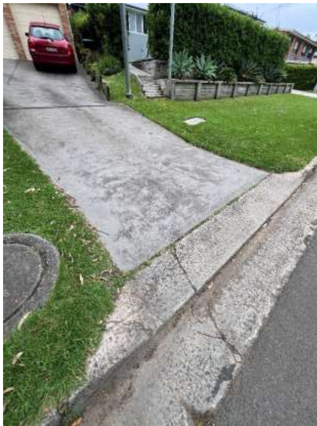
Figure 118 – Crack is evident to the layback outside 84 Warriewood Road Warriewood.
