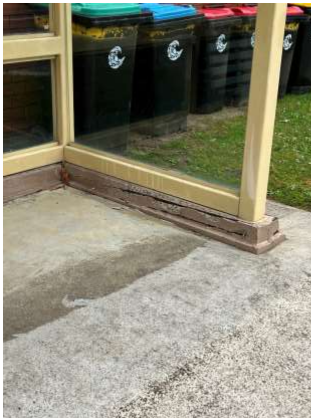
Figure 60 - Crack is evident to the concrete at bus stop outside 92 Warriewood Road Warriewood.
