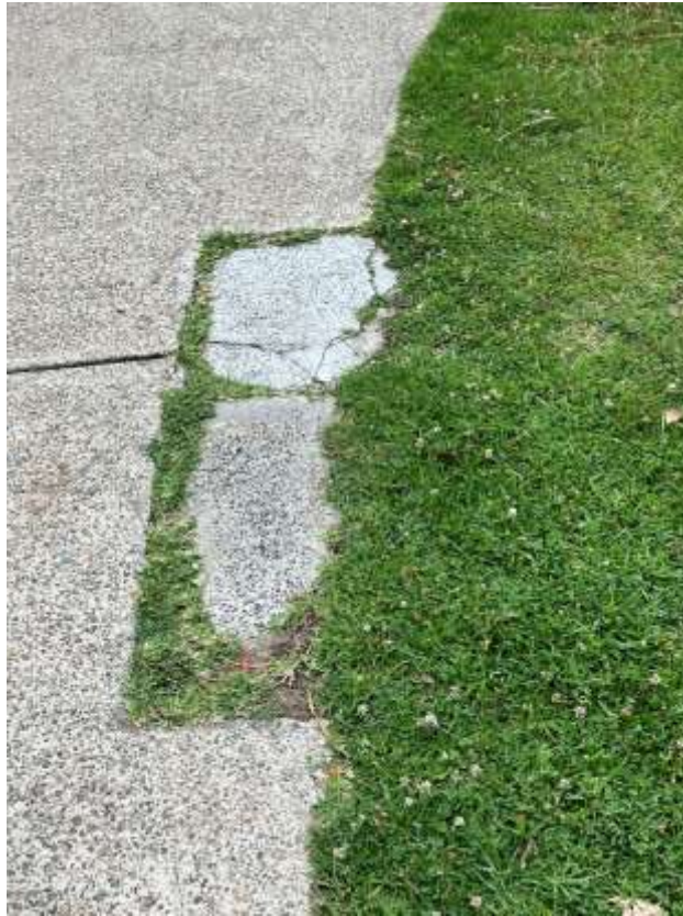
Figure 139 – Crack is evident to the pit outside 80 Warriewood Road Warriewood.
