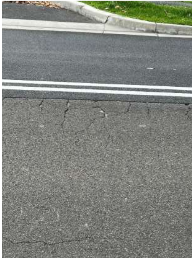
Figure 117 – Crack is evident to the road outside 84 Warriewood Road Warriewood.
