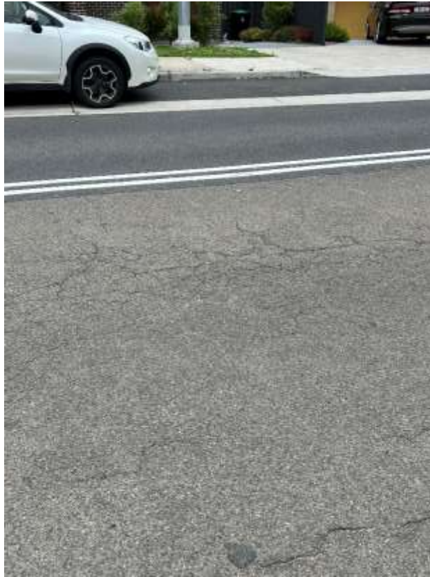
Figure 129 – Crack is evident to the road outside 82 Warriewood Road Warriewood.
