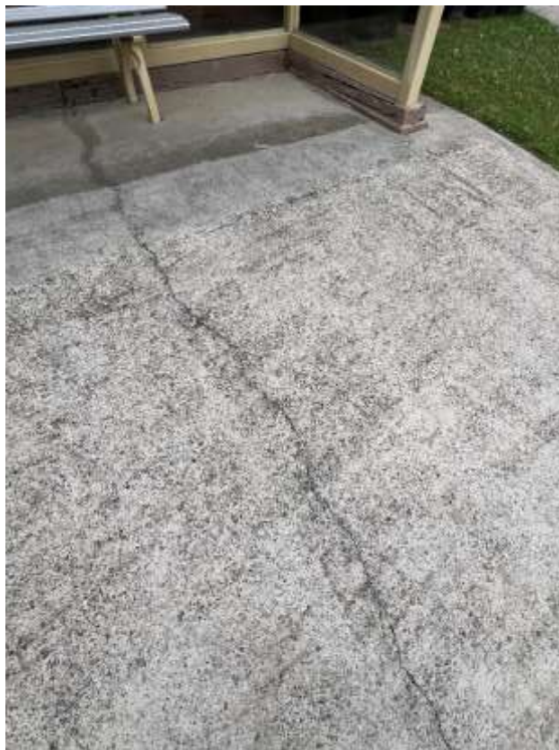
Figure 62 – Crack is evident to the concrete at bus stop outside 92 Warriewood Road Warriewood.
