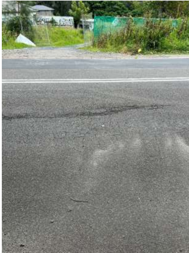
Figure 95 – Crack is evident to the road outside 86 Warriewood Road Warriewood.
