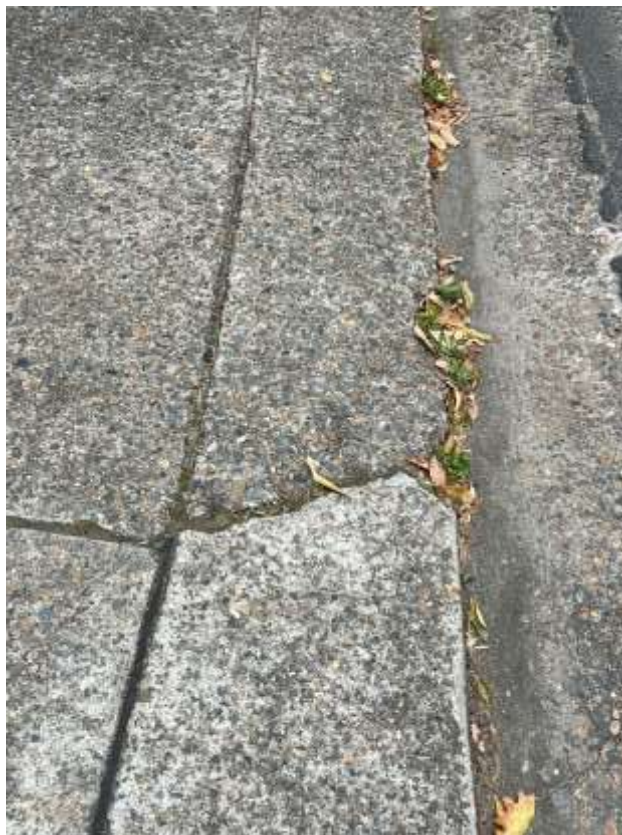
Figure 86 – Crack is evident to the layback outside 88 Warriewood Road Warriewood.
