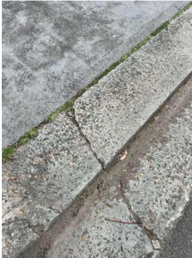
Figure 119 – Crack is evident to the layback outside 84 Warriewood Road Warriewood.
