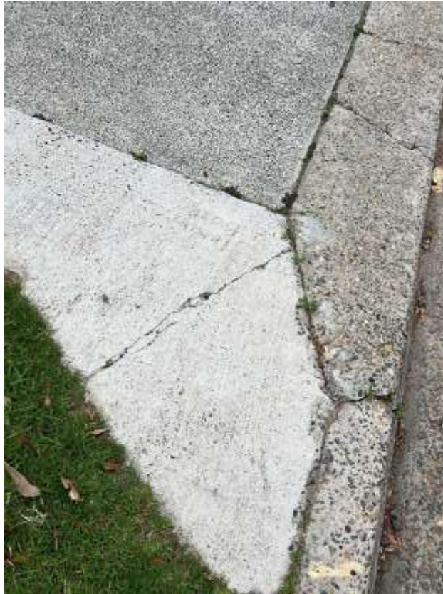
Figure 65 – Crack is evident to the layback outside 92 Warriewood Road Warriewood.
