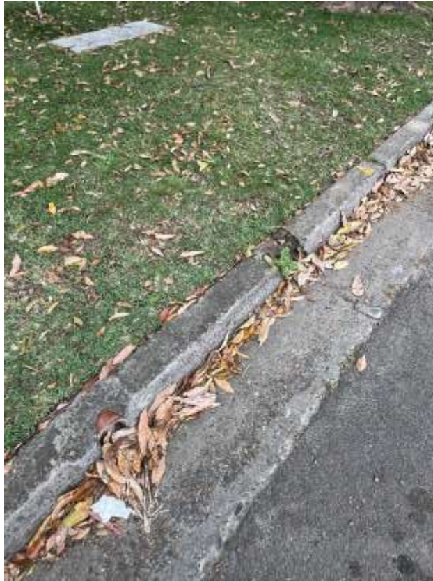
Figure 91 – Crack is evident to the kerb outside 86 Warriewood Road Warriewood.
