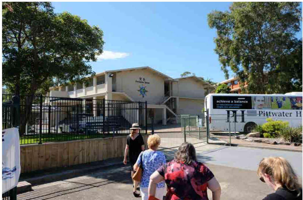
View north-east from the car park towards M Block.
