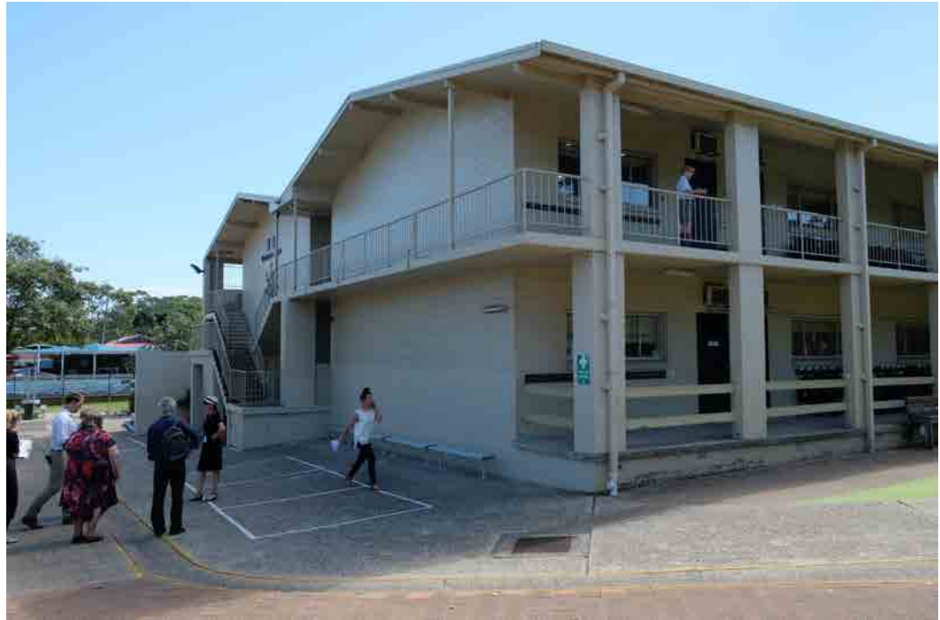
View north-east of M Block.
