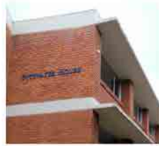
Face brick walls Painted concrete
