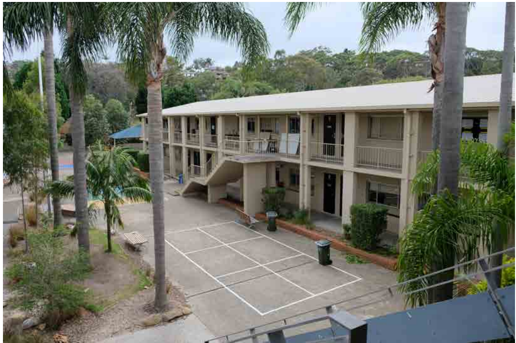
View north along M Block.
