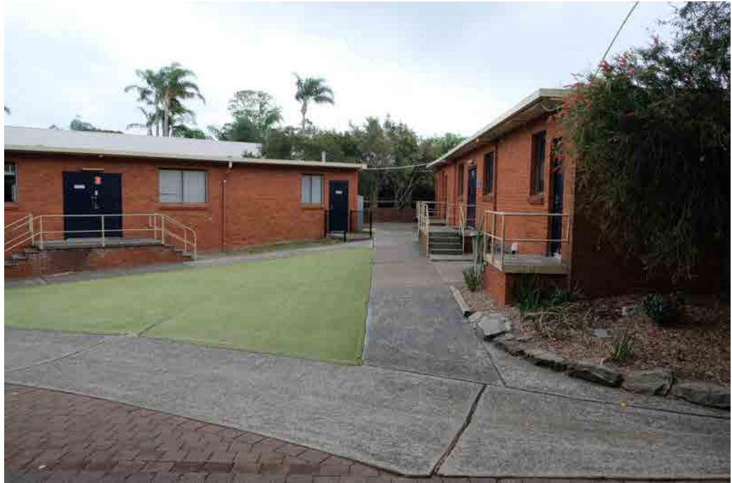
Ancillary demountable service buildings and sheds to be demolished.
