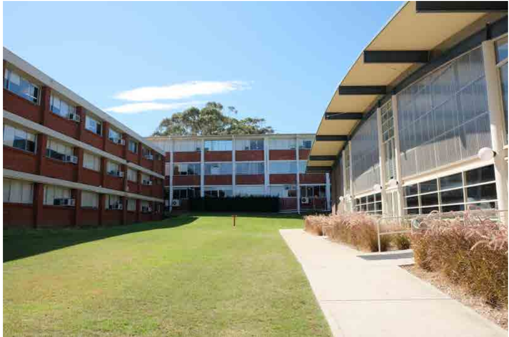
View north towards West Wing with the Sports Hall to the right and South Wing to the left.
