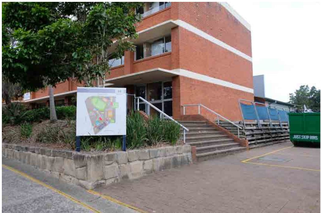
View of south-wing looking north.
