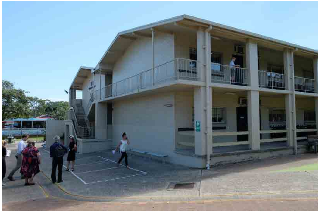
View north-east of M Block.
