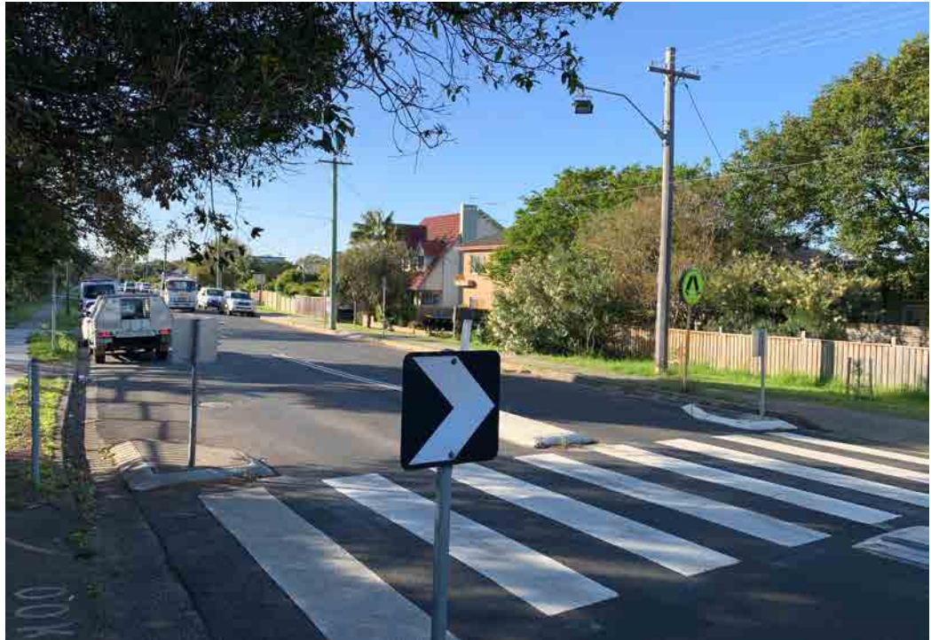
Existing pedestrian crossing on South Creek Road.
