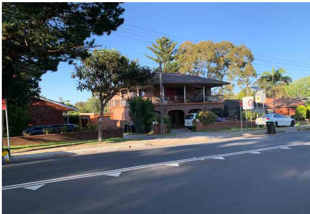
View south-west of 63 - 67 South Creek Road
