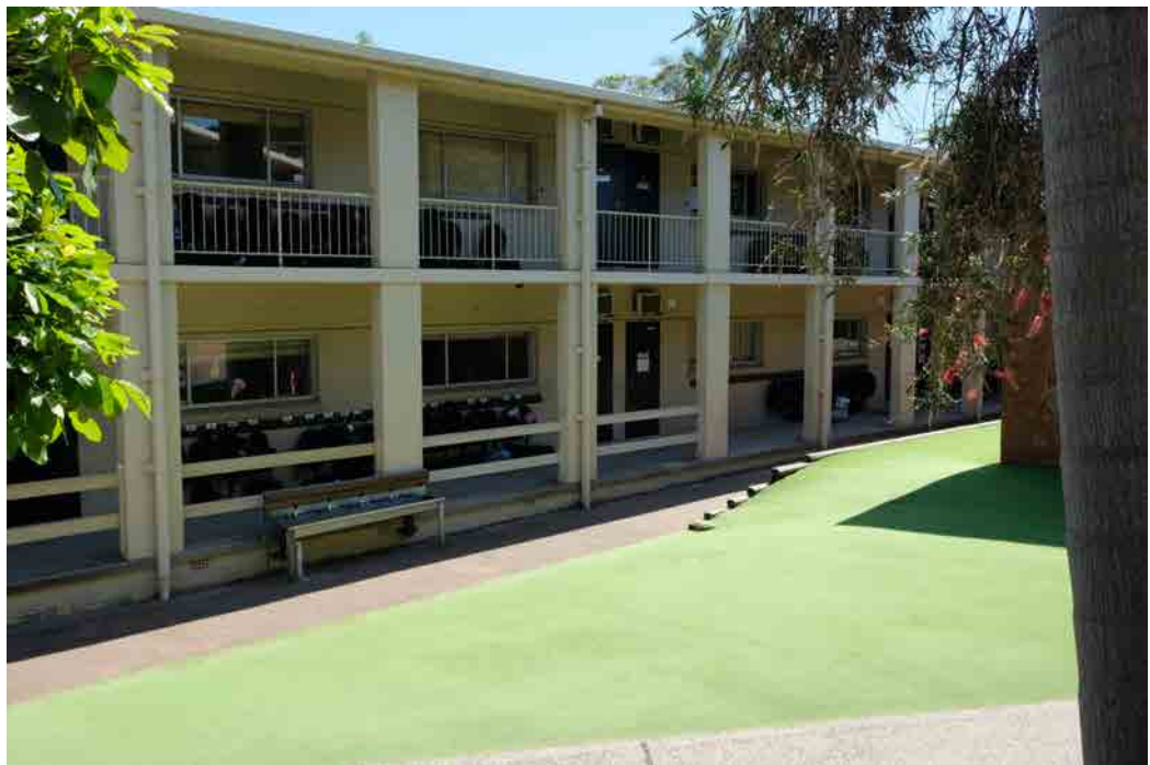
View south to South-Wing.
