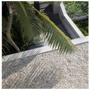
GR GRAVEL BALLASTED ROOF
