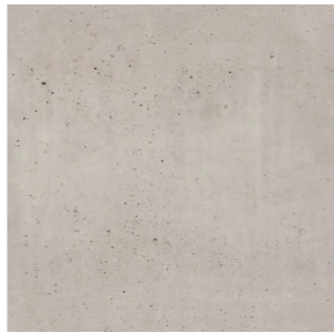
CONC NATURAL OFF-FORM CONCRETE
