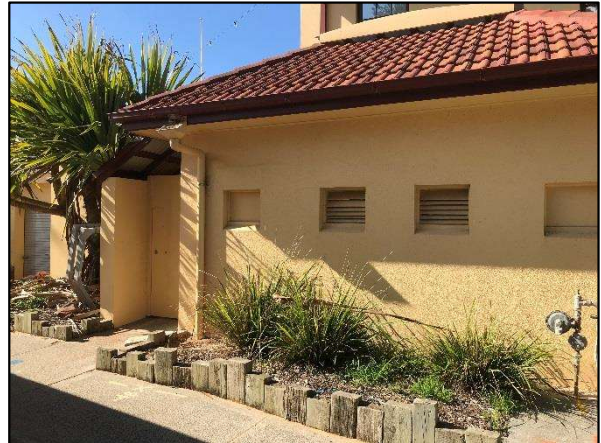
Figure 53. View of the northern wing and side wall that may leads may have led to an earlier entrance to change rooms. (Source: Heritage 21, 23.05.18)
