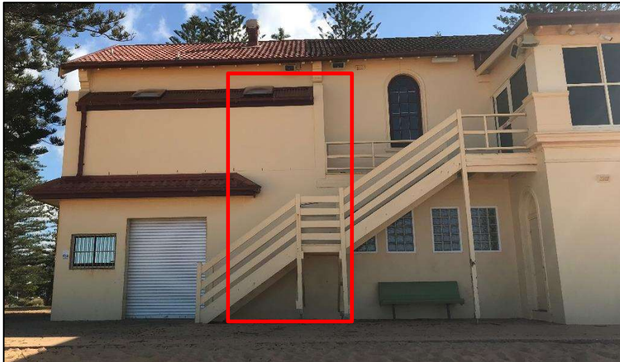
Figure 108. Current alignment of wing and central section walls.
