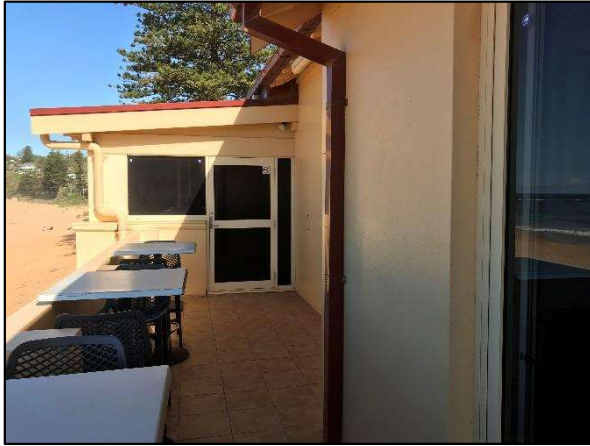
Figure 104. View of the open to sky terrace extended east from the Northern Wing. Note enclosed veranda extension behind the seating area. (Source: Heritage 21, 23.05.18)
