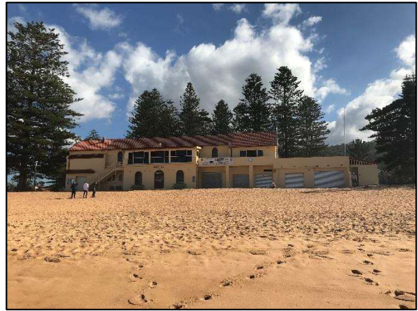
Figure 57. View of the eastern elevation as seen from Newport beach. (Source: Heritage 21, 23.05.18)
