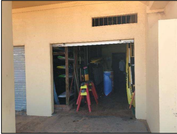
Figure 82. Storage areas with roll-up shutter doors. (Source: Heritage 21, 23.05.18)
