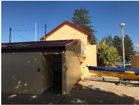
Figure 60. View to the entrance of the female public toilets along the northern skillion lean to. (Source: Heritage 21, 23.05.18)
