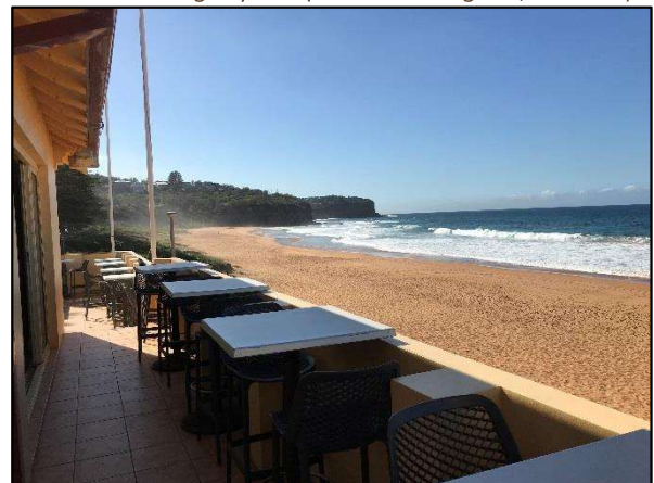
Figure 103. View of the open terrace extended beyond northern wing looking towards the main beach. (Source: Heritage 21, 23.05.18)
