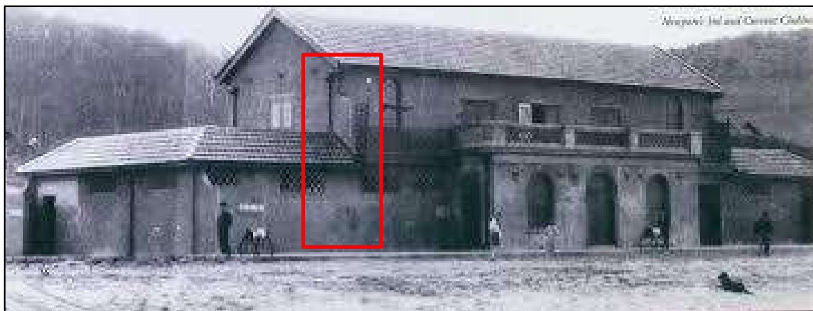
Figure 107. Photograph indicating original single storey wing alignment with two-storey section walls
