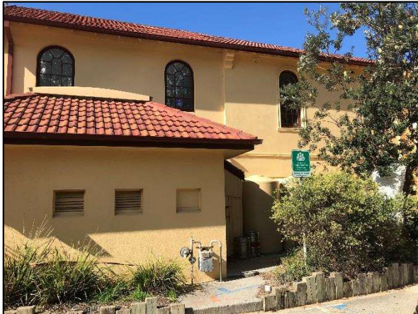
Figure 52. View of the Northern wing. Note the recessed wall between the original and the later addition northern extension. (Source: Heritage 21, 23.05.18)
