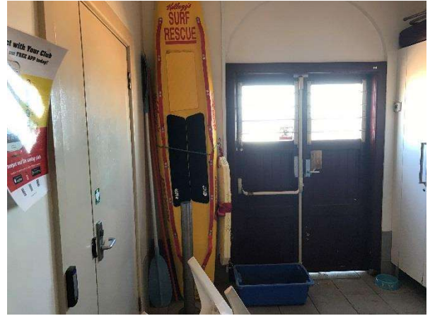
Figure 73. Exit Door to beach. (Source: Heritage 21, 23.05.18)
