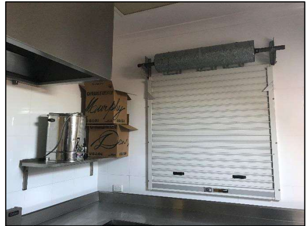
Figure 99. Service window from kitchen that opens into the main club room. The door can be viewed on the club room end in Figure 48. (Source: Heritage 21, 23.05.18)
