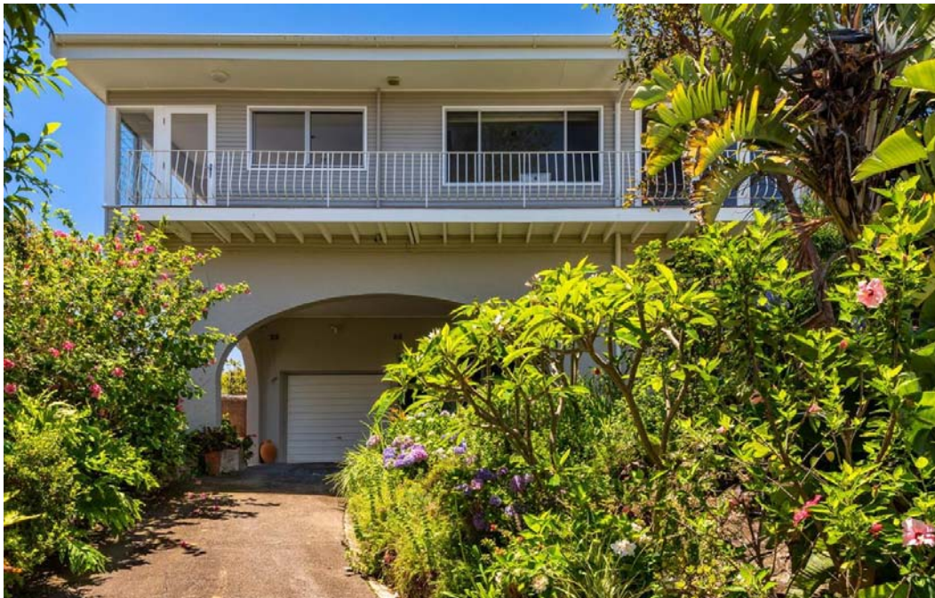
Photograph of the existing parking arrangements
