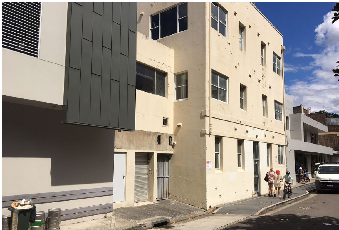
FIGURE 4a Existing Market Lane Loading Zone (view west)
