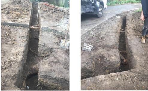
Figure 2 and 3: Exposed trenches and roots.
