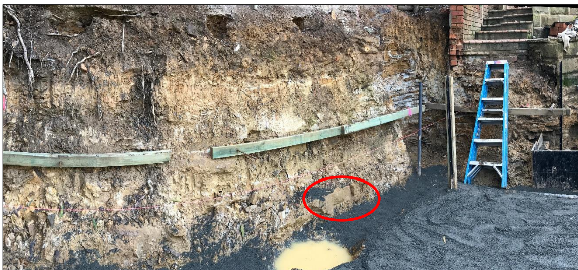
Photograph 7: View of the front of the excavation adjacent No.67 Dolphin Crescent with an interbed of competent bedrock (circled red).
