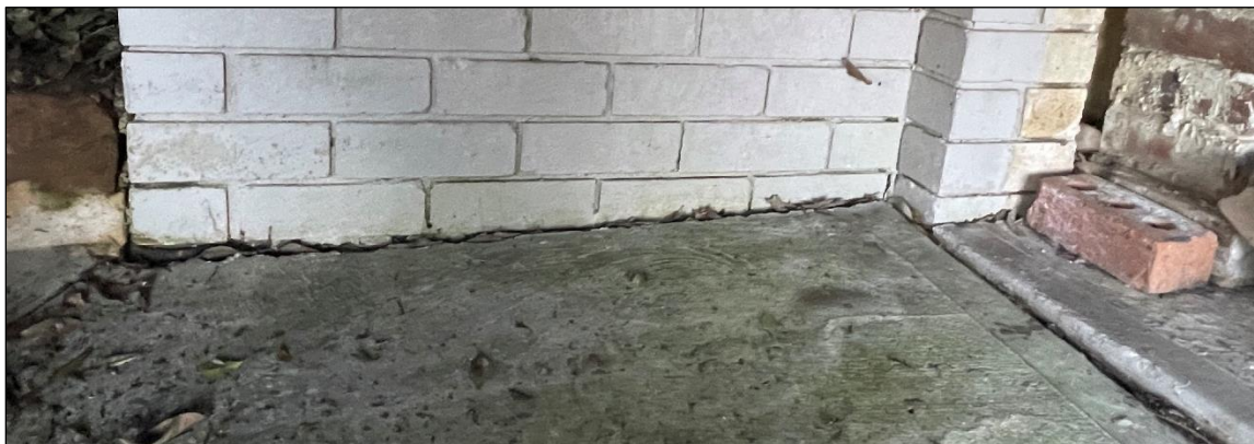
Photograph 6: Gap between concrete slab and external wall of the dwelling
