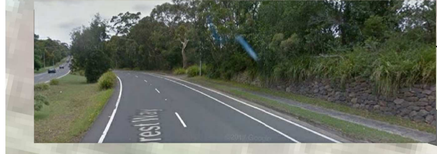
VIEW LOOKING NORTH UP FOREST WAY ALONG SITE
