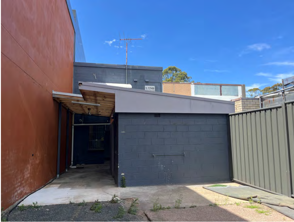
Photograph 4: Rear of 1749 Pittwater Road
