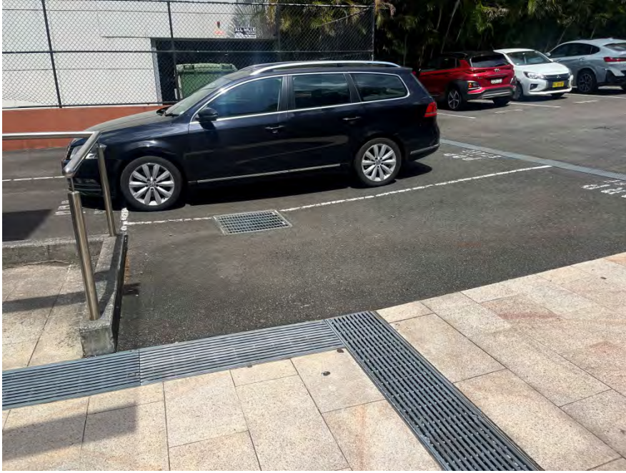
Photograph 3: Rear of 1753 Pittwater Road
