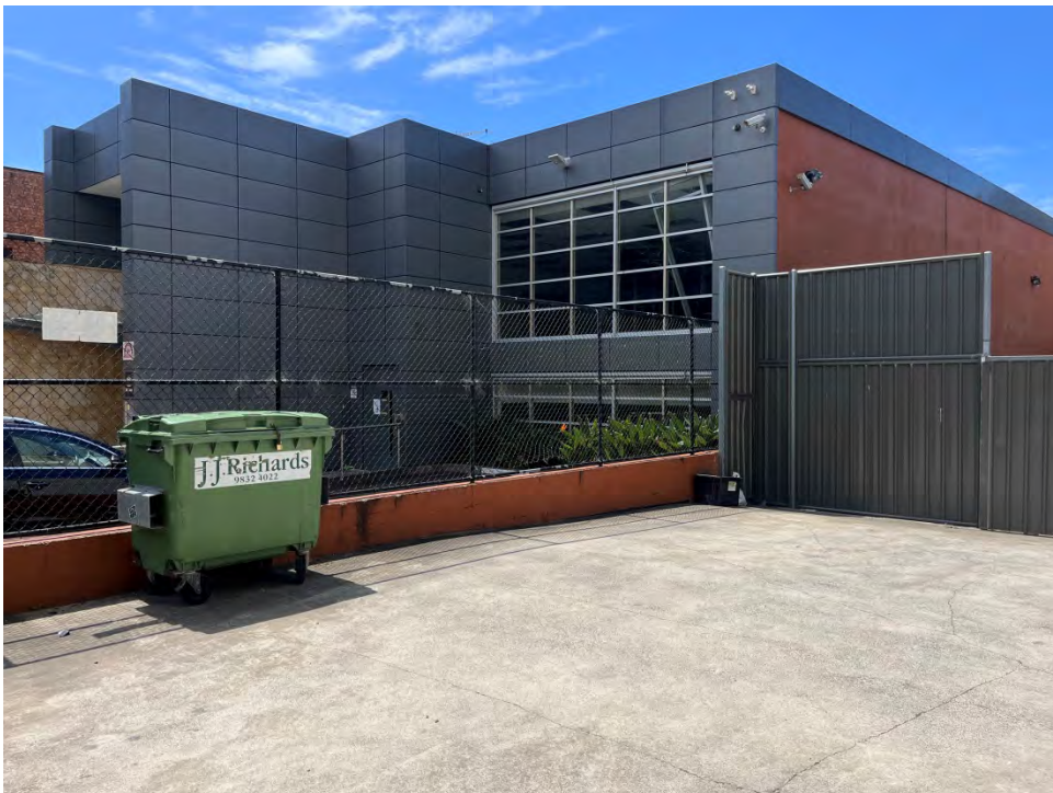
Photograph 4: Rear of 1749 Pittwater Road
