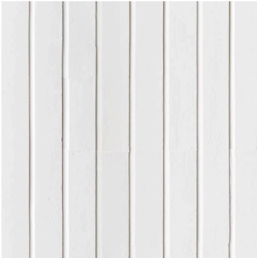
Weatherboard Cladding - new works - white paint finish to match existing
