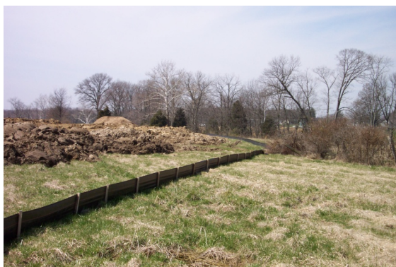
Example – Silt Fencing
