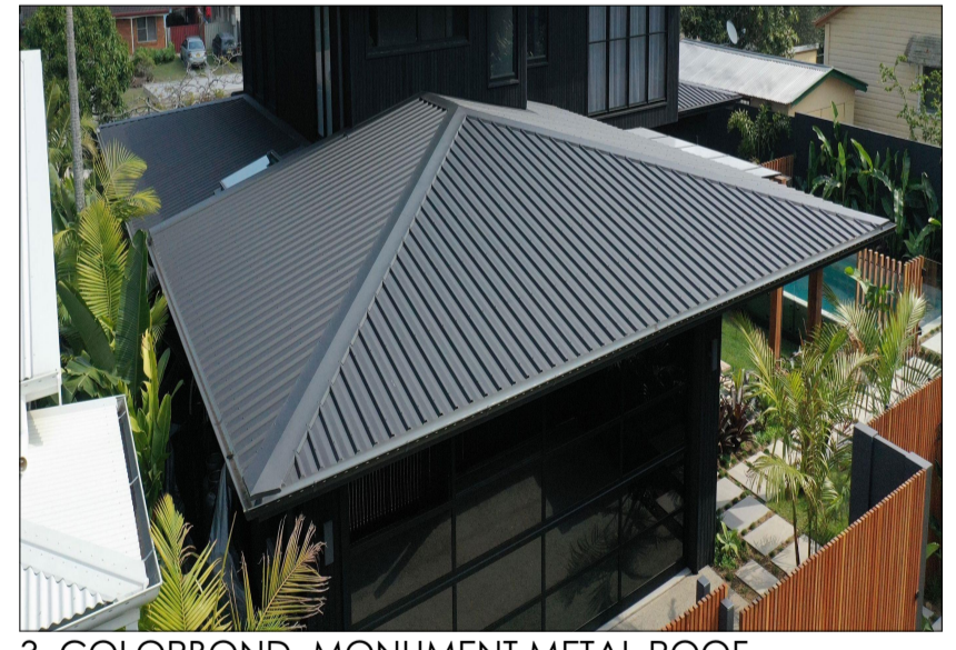
3. COLORBOND MONUMENT METAL ROOF
