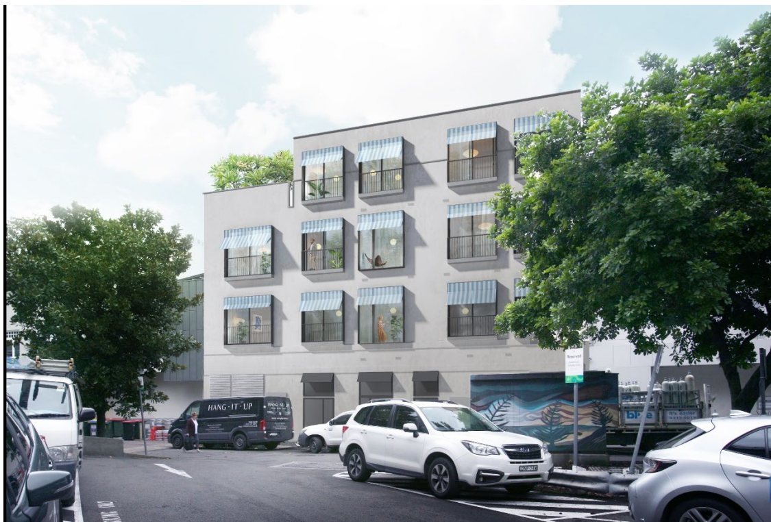
Photograph 3: Market Lane frontage of the proposed development, demonstrating the overall facade composition, including that part of the building which is non-compliant with the development standard
