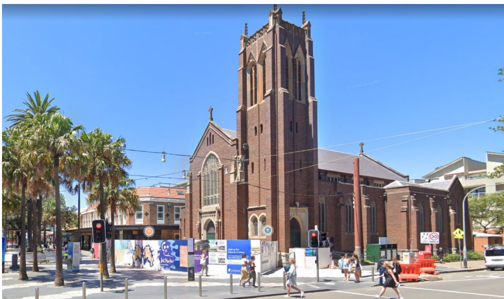
Figure 2: St Matthews Manly, located on the southern side of The Corso, opposite the site, at 1 Darley Road
