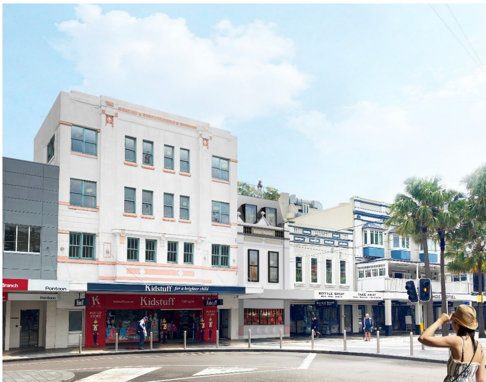
Photograph 1: View looking north-east towards the subject site, demonstrating how the proposed form above No. 23 sits with the built form directly east and west of the buildings comprising the site
