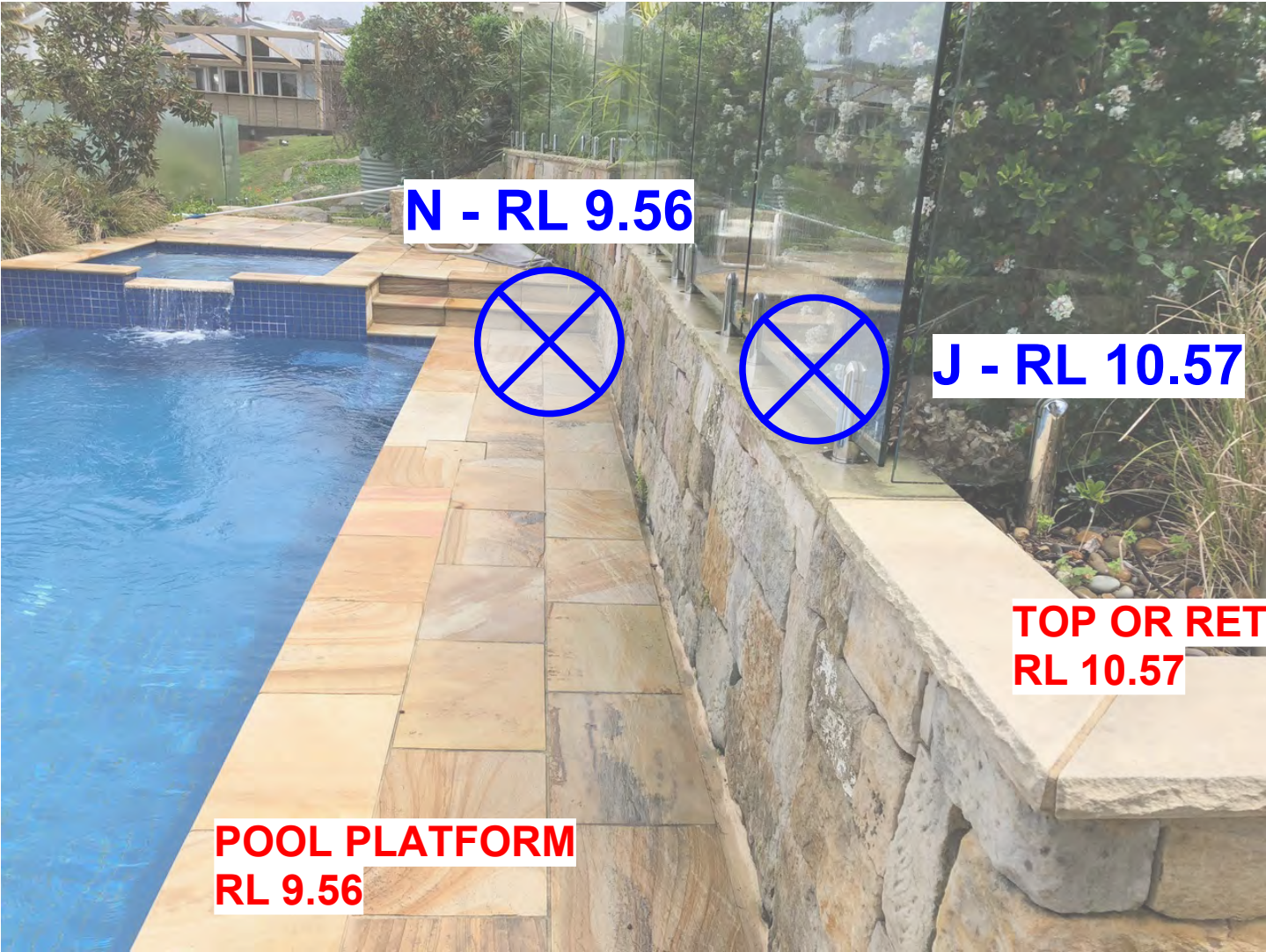
Photo of existing pool, stone retaining walls and garden terraces. Edited by VK showing points's location and relative levels.
