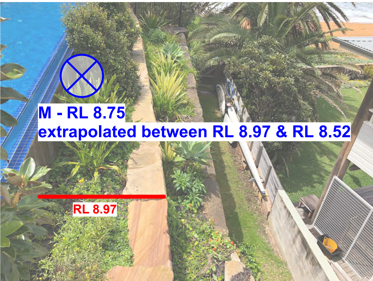
Photo of existing pool, stone retaining walls and garden terraces. Edited by VK showing points's location and relative levels.
