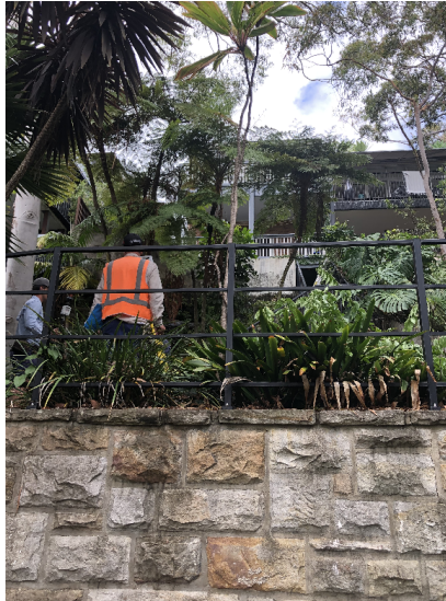
SANDSTONE FACED RETAINING WALL
