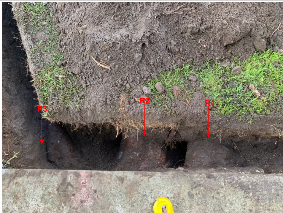
Image 4: Looking South within root investigation trench 1, showing root 1, 2 and 3.
