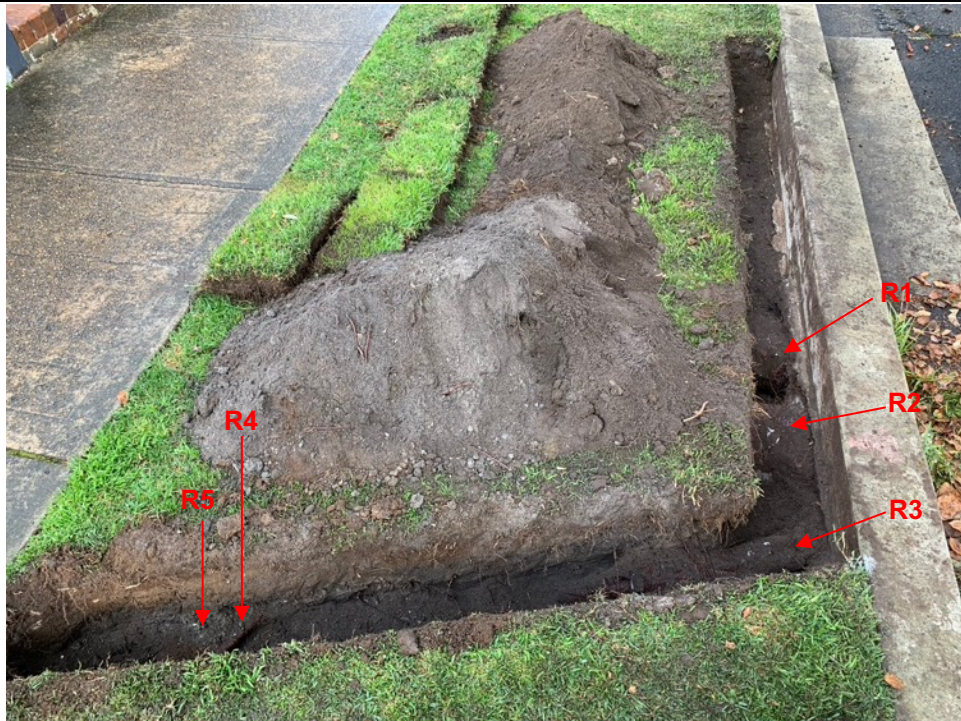
Image 3: Looking West towards root investigation trench 1, showing the location of roots 1, 2, 3, 4 and 5.
