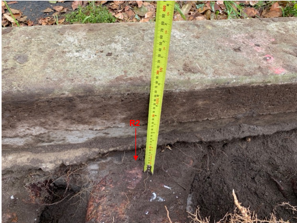
Image 11: Looking North within trench 1, showing the depth of root 2 (270mm below existing grade).
