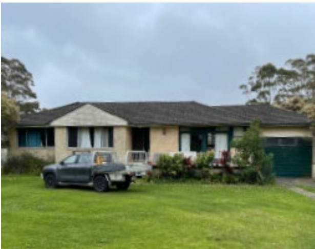
Picture 5 Existing residence on site
