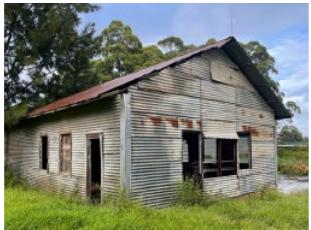
Picture 4 Existing building on site
