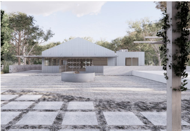
Picture 15 restaurant 1 viewed from outdoor dining terrace
