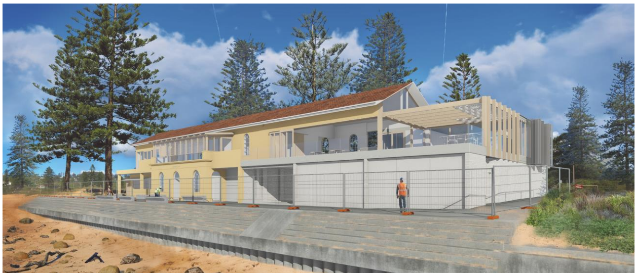
Figure 4: Photomontage of proposed works (with piling exposed) as may temporarily occur after severe storm erosion which requires beach closure, until sand levels are naturally restored, or this process is mechanically accelerated by Council undertaking beach scraping. A temporary solid barrier may also be employed to reduce wave forces on the clubhouse, see Horton Coastal Engineering (2021)
