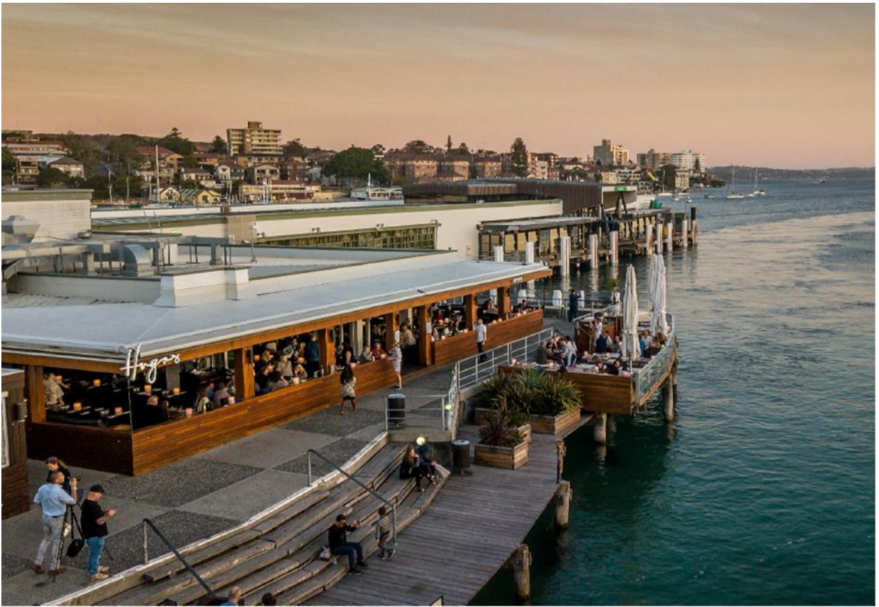
Figure 4 - Photo of the existing site (Squillace Architects)
