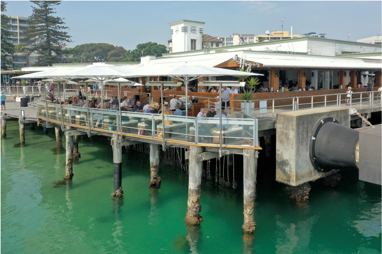
Figure 5 - Photo of the current seating area (Squillace Architects)
