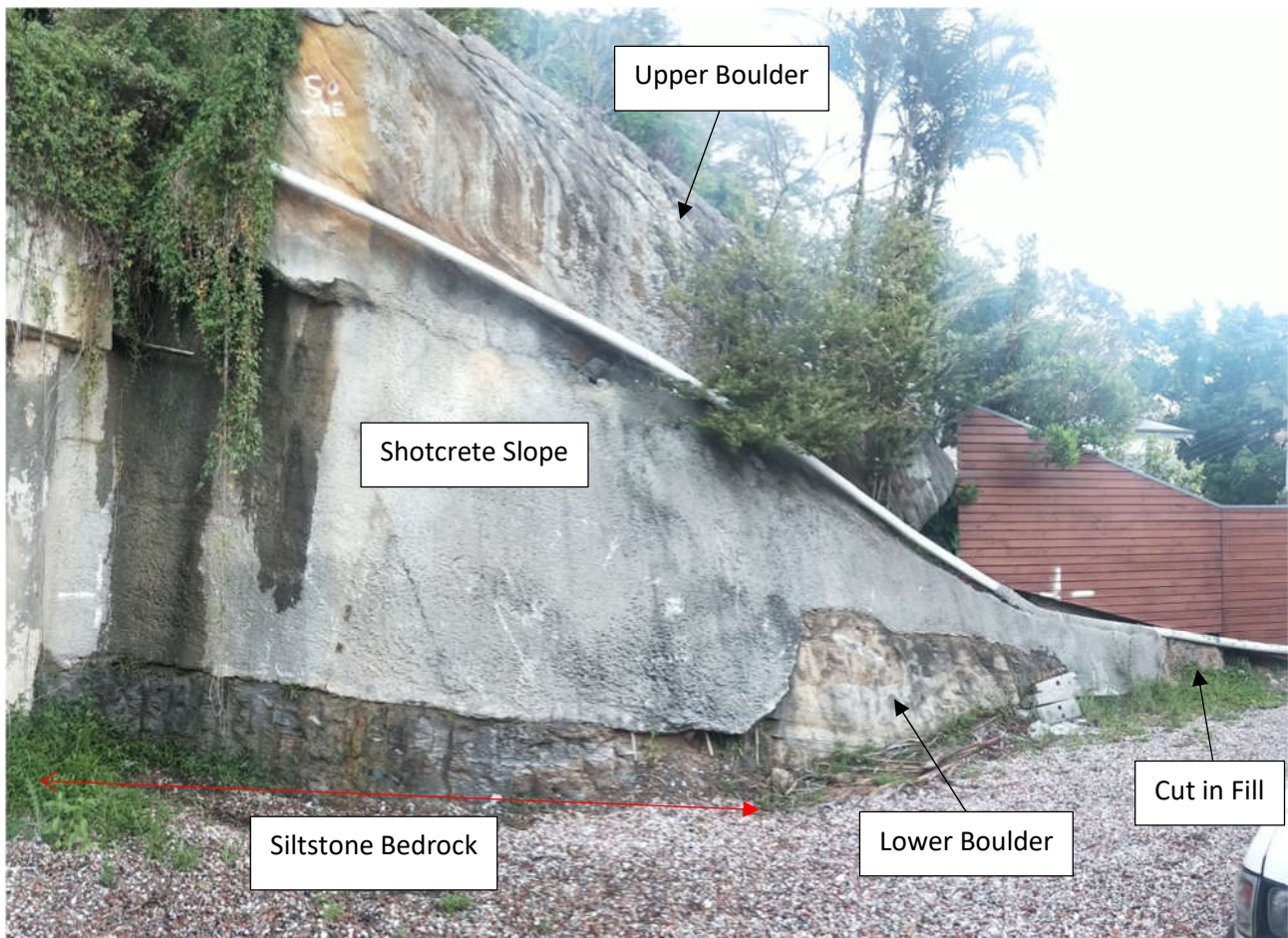
Plate 2: Photograph 1 of Large Boulders and Shotcreted Cut Face At/Near Southern Boundary (Facing South)
