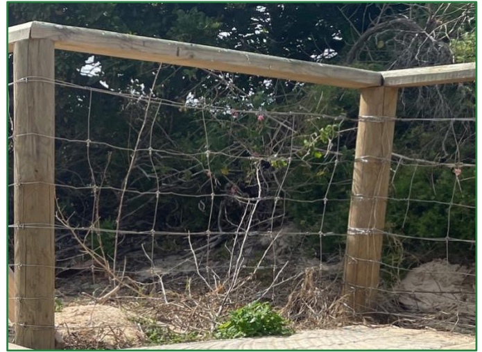
Photo 2. Stainless steel wire mesh attached to timber fence
