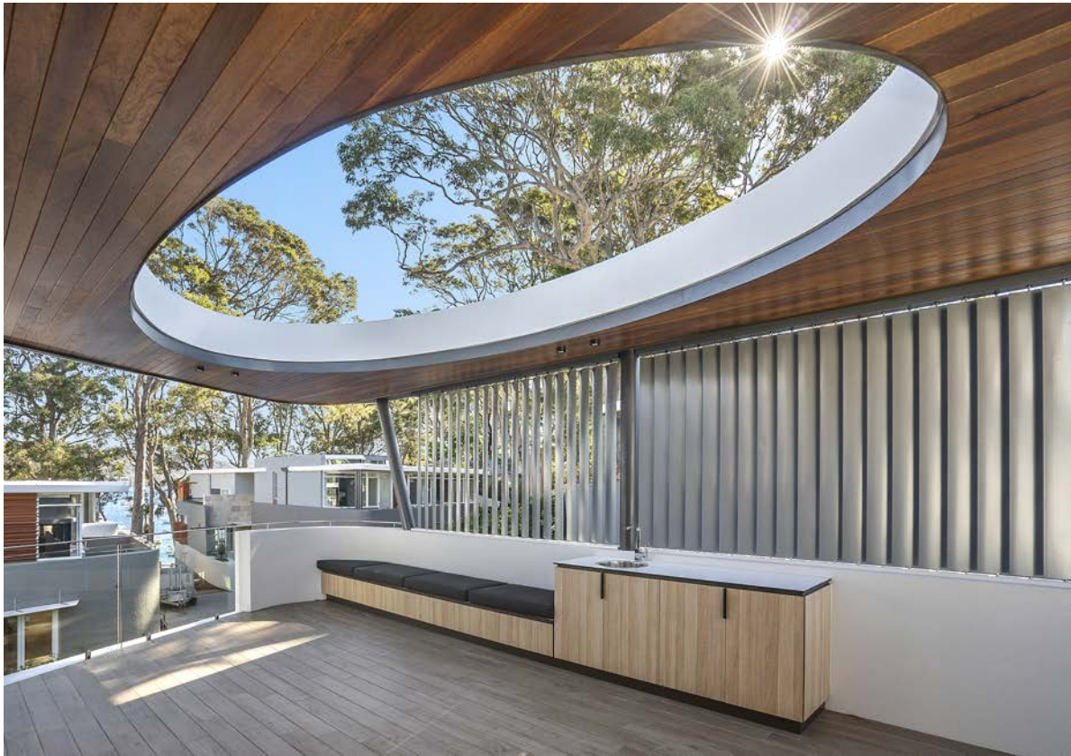
1 PROPOSED PRIVACY SCREENS ADJUSTABLE VERTICAL BLADES
