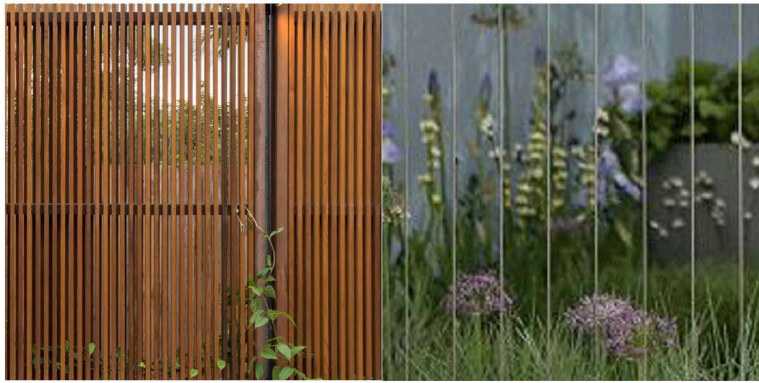
7 TIMBER BATTENS AND STEEL CABLE WIRES
