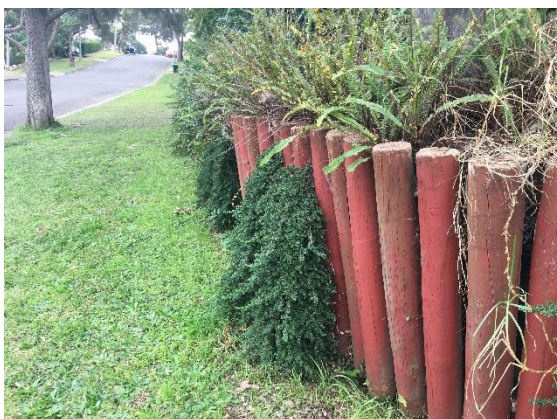
Photograph: 5 □ Timber log retaining wall west bdy.
