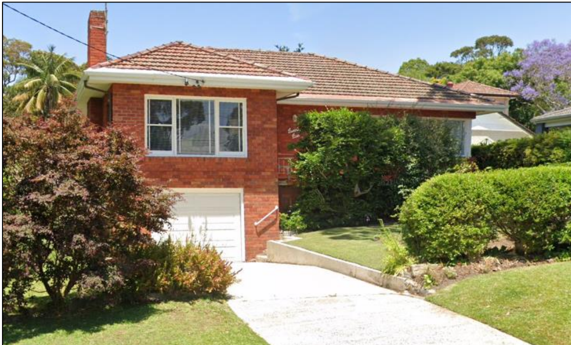
Figure 02: Subject Site at No. 25 Valley Road, Balgowlah Heights (Google Maps, accessed 2024)
