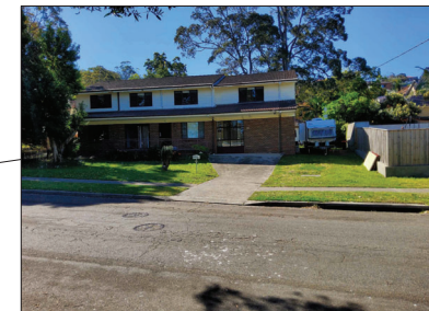
EXISTING DRIVEWAY AND EXISTING BUILDING, TO BE DEMOLISHED FOR PROPOSED DRIVEWAY AND HARDSTAND AREA
