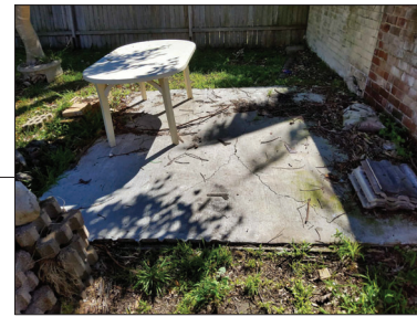
EXISTING CONDITION OF COUNCIL DRAINAGE ASSET TO BE RETAINED
