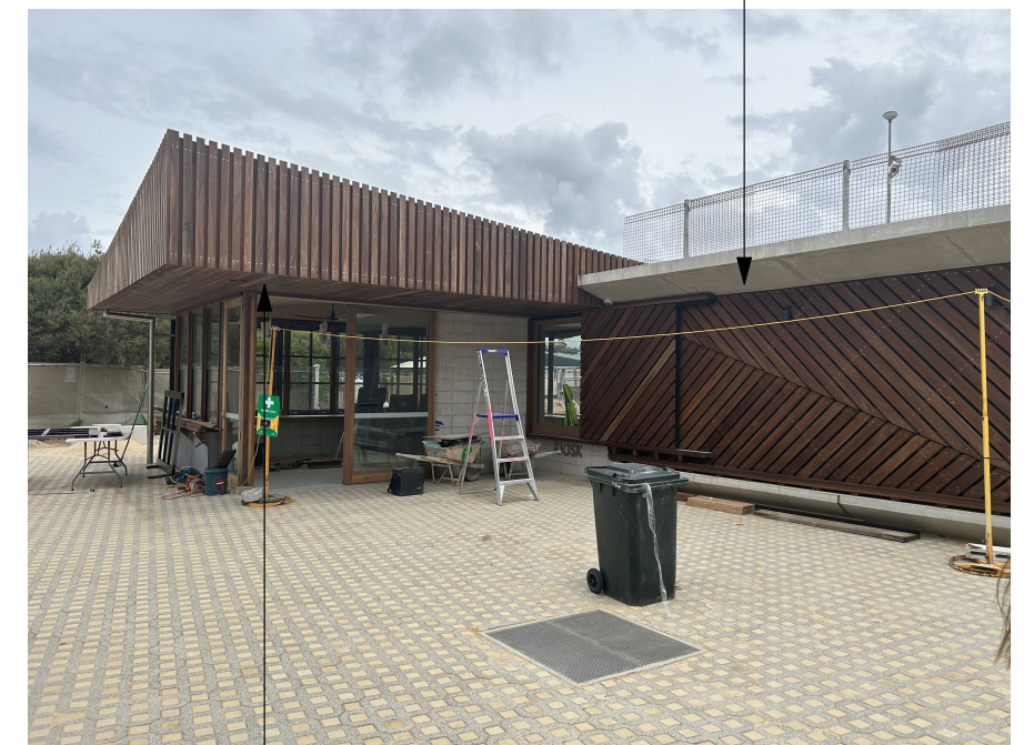
EXISTING TIMBER CLAD EAVE OVER TENANCY
