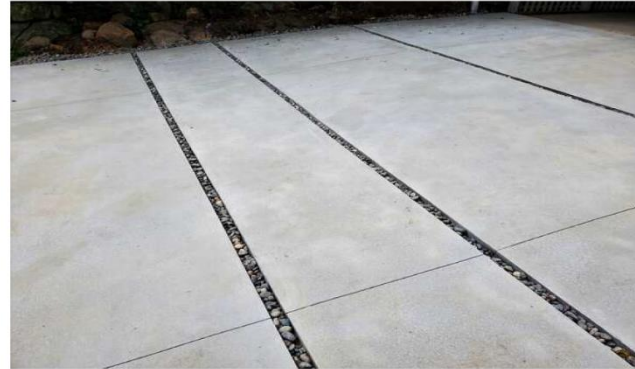
Driveway - Sandblast concrete with gap between slabs
