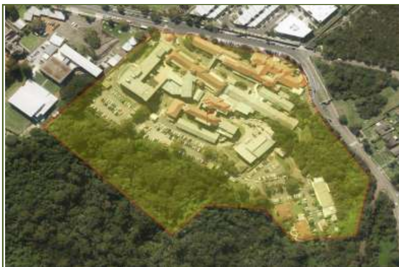
Figure 1.2: Existing condition of the land (Google Maps 2018)
