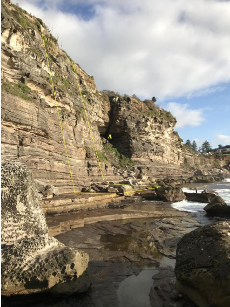
Figure 4: View of cliff face and rock platform at subject property on 7 April 2018, looking NW, with approximate lot boundary depicted, and St Michaels Cave visible in background at "A"
