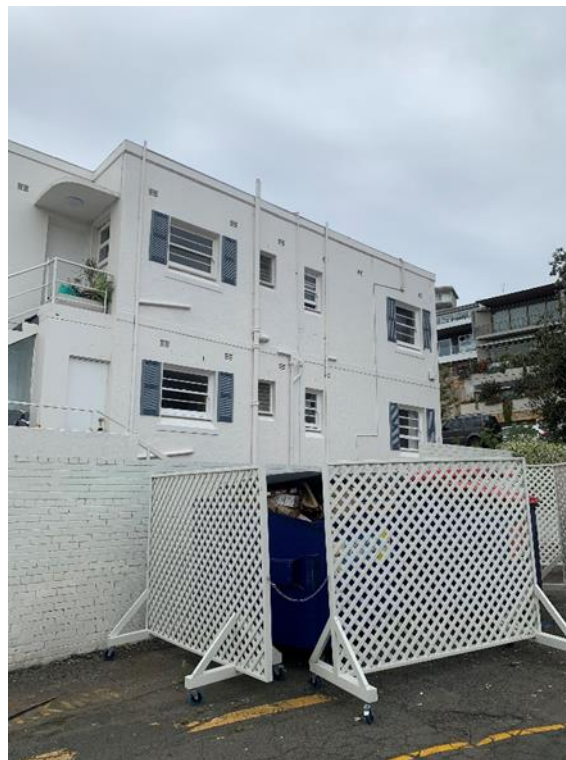
Figure 13. The current hotel and carpark. The slope of the study area is partly visible.
