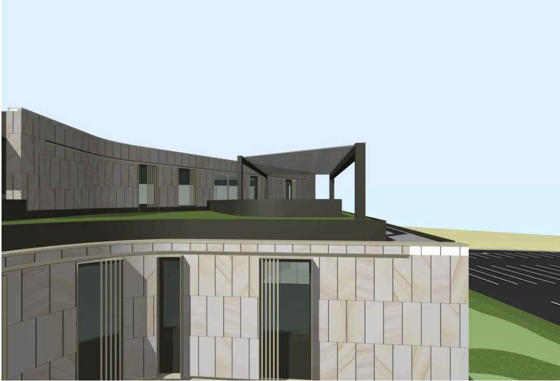
Image 7: Building E with proposed awning on Level 4, SE side. Awning fully extended.
