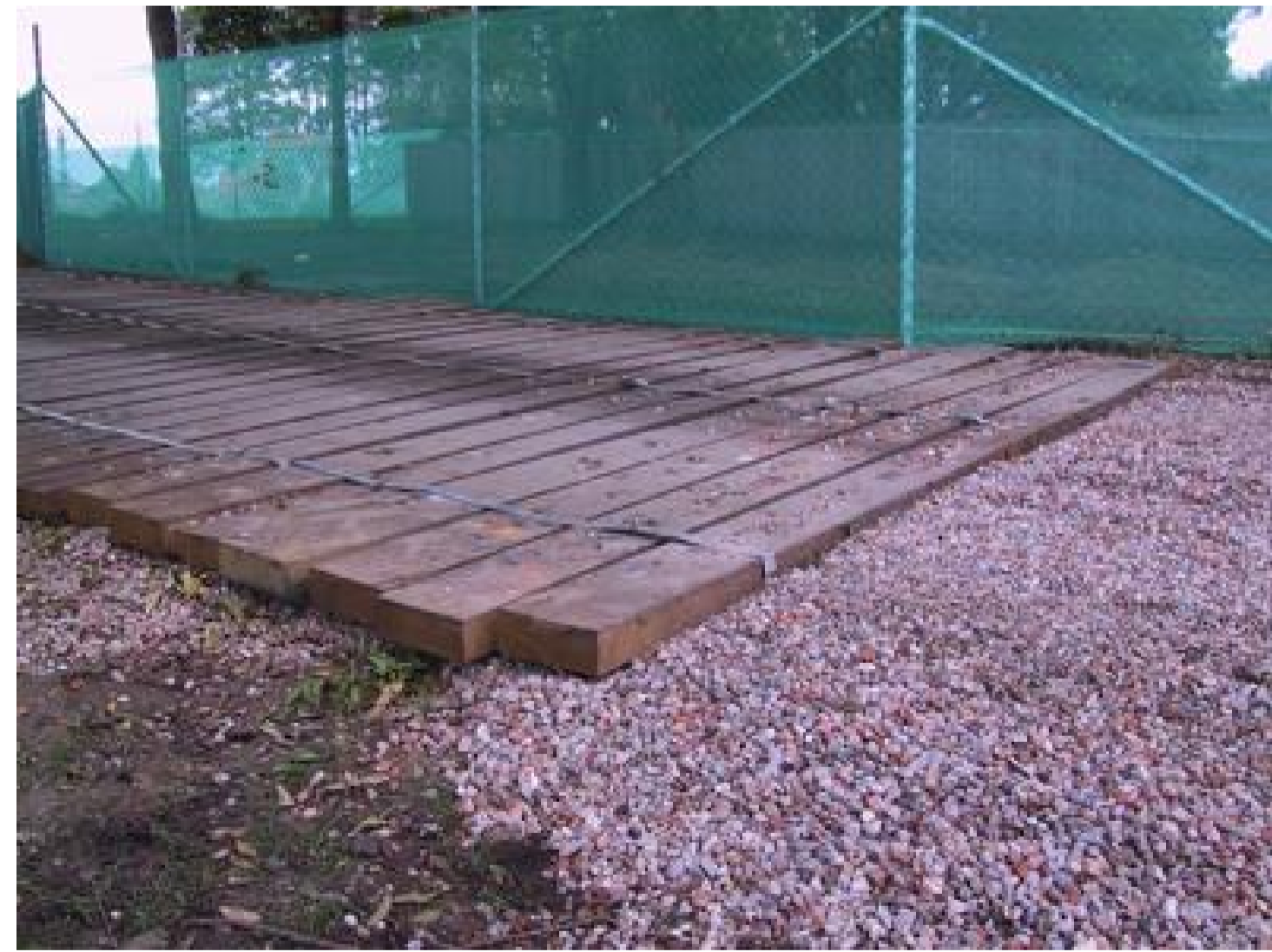
Example image of acceptable ground protection rumble boards
