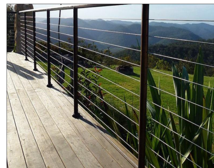
all balustrades rendered blockwork steel wire balustrade
