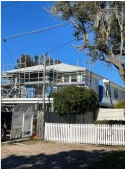
9 Lido Ave. currently under construction June 2024
