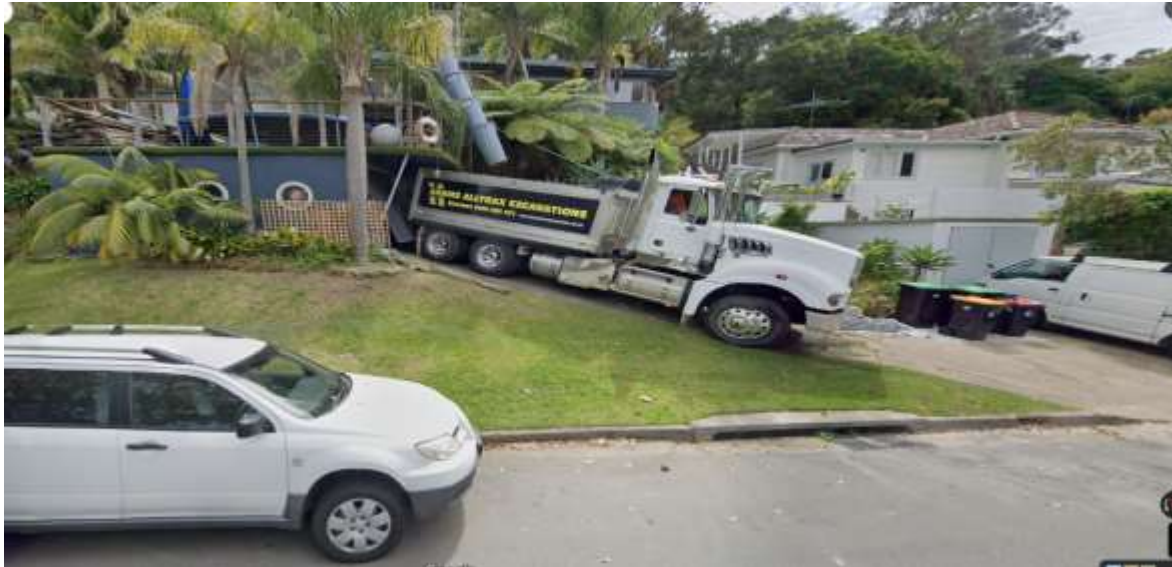
Number 14 blue double garage above porthole windows street side wall Number 12 single white garage and house right side photo.
