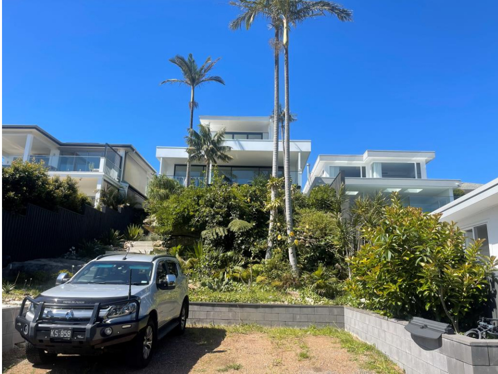
Fig 2: View of subject site, looking south from Bushey Place
