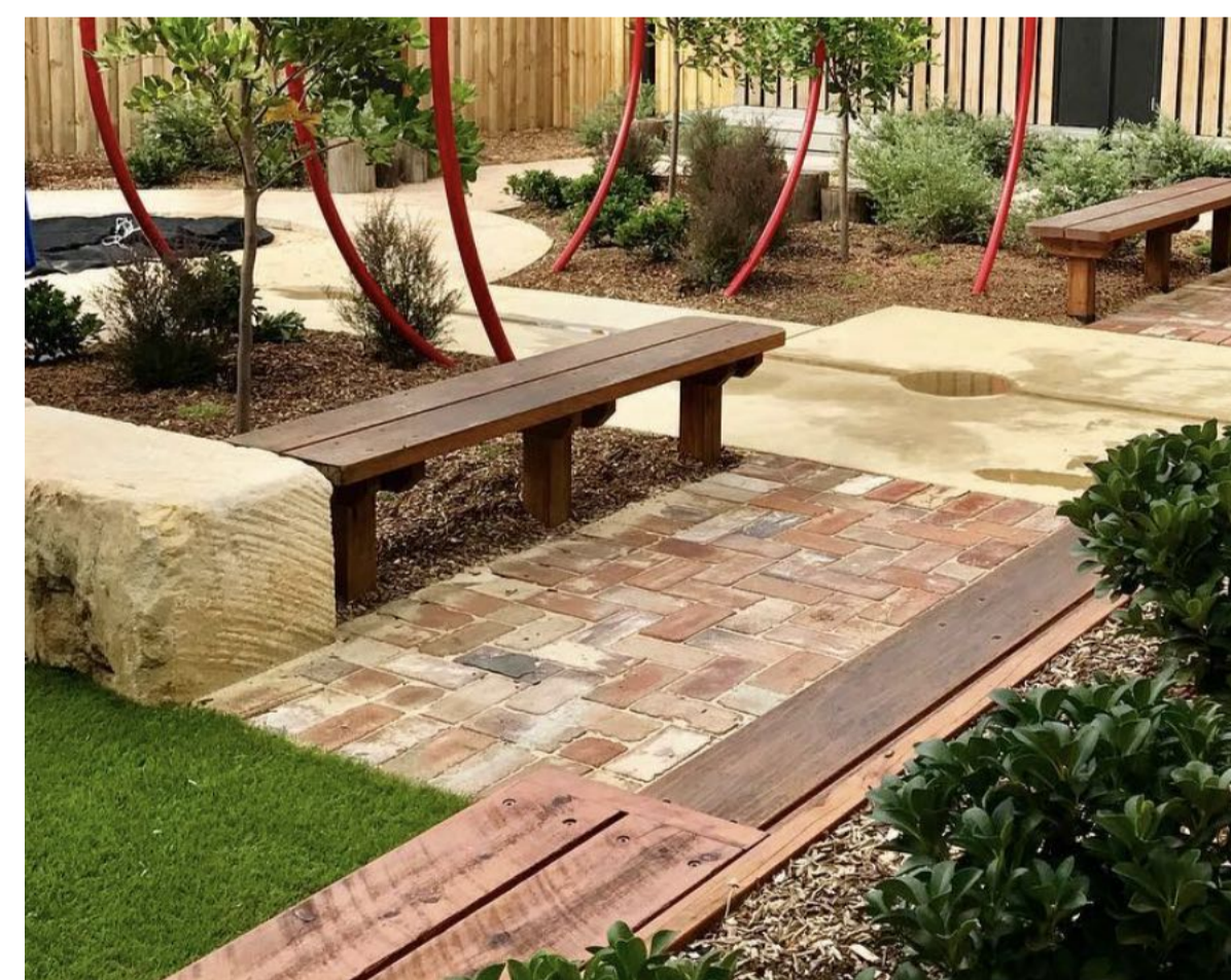
Recycled brick Paving
