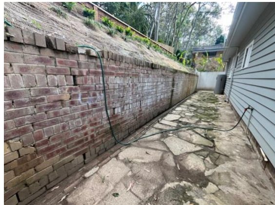
Photo 4: Brick wall at dwelling rear
